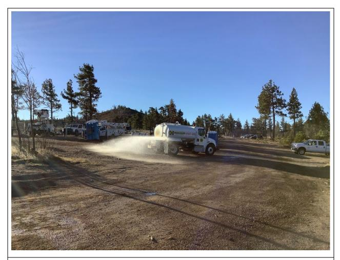
**Photo 1:** A water tender was observed applying water to the surface at Shrine Camp Staging Yard (C 440) throughout the day to minimize dust emissions in accordance with APM AIR-02.
