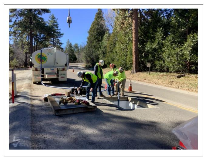
**Photo 6:** During dewatering at a hand hole along Sunrise Highway (C 440), water was pumped into a truck-mounted storage tank for dispersal in accordance with APM HYD-08.
